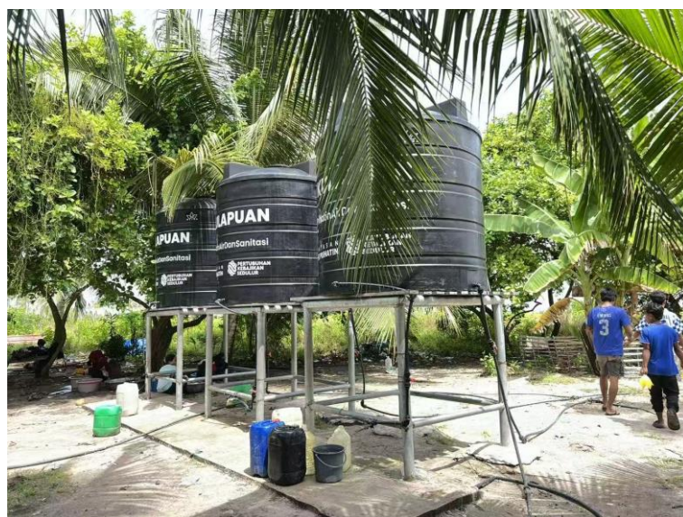
Figure 1. Community Water Supply Facilities: Water Tower and Pump System. Source: Photo by the Author during Fieldwork, February 12, 2026.
