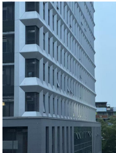
Figure 1. Chongqing University of Education Main Teaching Building(China)
